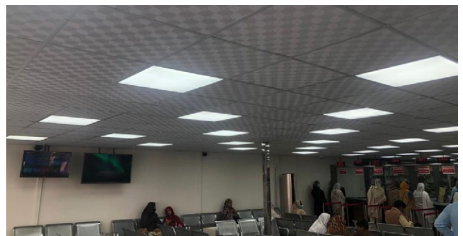
Picture 9: Replacement LED panels in the reception area
