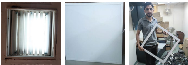
Picture 4. Original 26 inch x 28 inch recessed fluorescent tube luminaire (left), 24 inch x 24 inch LED planar (centre) and its frame (right).
