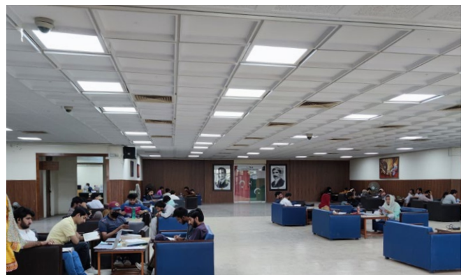
Picture 5. The lower entrance floor of QUA Library Building before (left) and after (right) the installation of replacement LED luminaires
