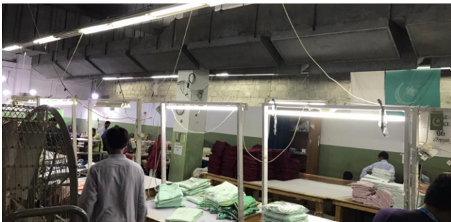
Image Pakistan Ltd replaced the 890 existing fluorescent tubes in their production lines with LED tubes
