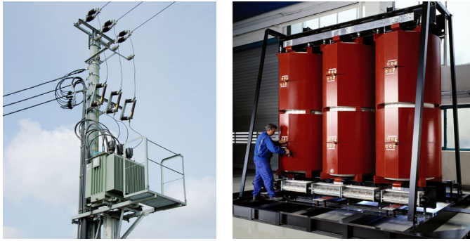
Typical liquid-filled (left) and dry-type (right) transformers
